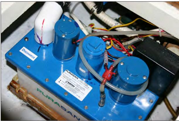
A few weeks ago I noticed slight leakage of discharge seeping from the top of the Purasan treatment box. The leak was traced to a small slot at the base of the macerator motor on top of the second (discharge) chamber. Great, just what I needed. Time to repair the treatment tank!
