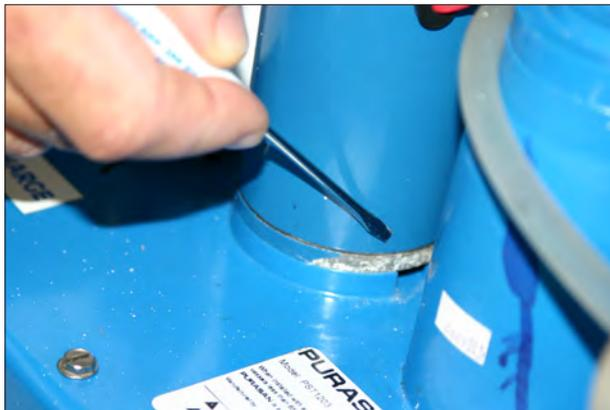
The Purasan treatment tank utilizes two chambers, an entry chamber and a discharge chamber. Each chamber has a macerator mixer motor mounted on top of the treatment box. The macerator motor spins a shaft that enters the treatment chamber and is protected by special seals manufactured by Raritan. Two seals cost about \$40 plus shipping from Raritan. Raritan part # 31-102, motor shaft seal.
